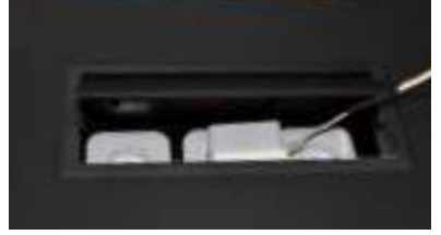
Cable Management Access
